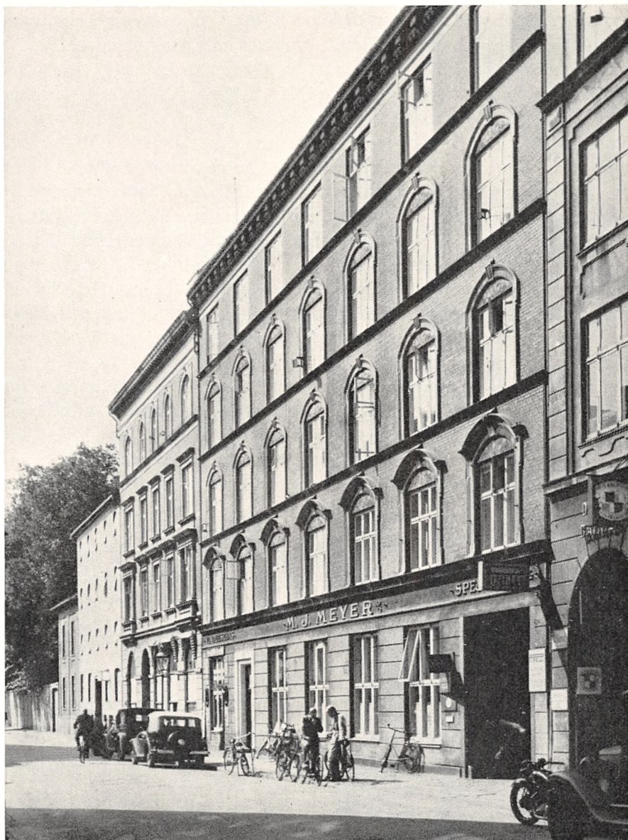
M. I. Meyer A/S's Administrationsbygning.
