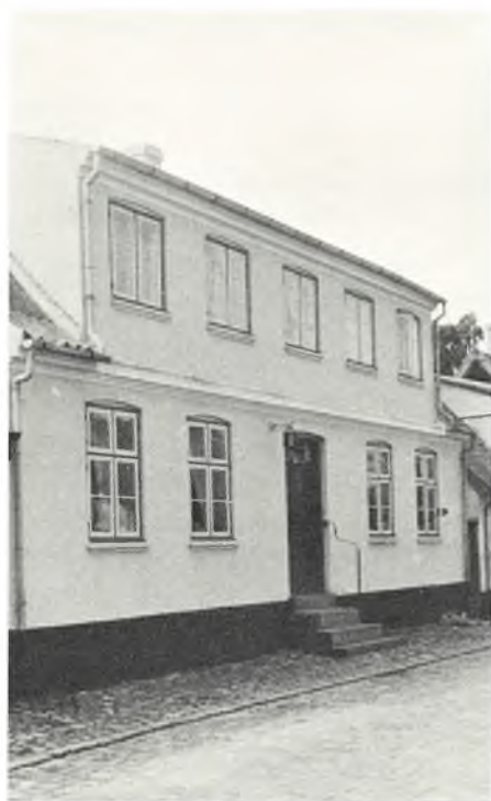
Strandgade 9, nordfacade. (NM 1977).
