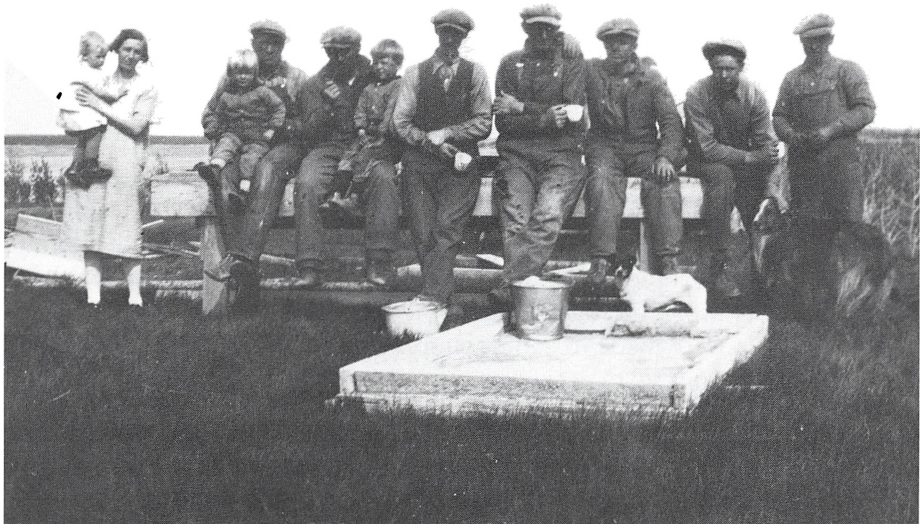
Digging the foundation of Dalum church. Summer, 1929.
